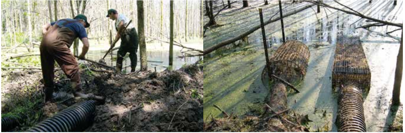
Figure 24.3 Beaver baffle control system
